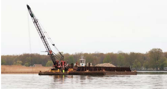
Crane and clamshell rock placement
