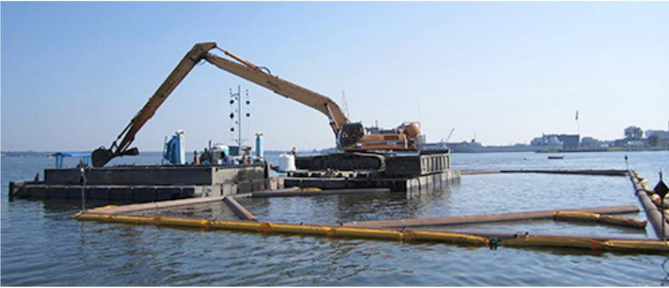
*Dredging with booms and screens to contain suspended sediment. Dredged material must be properly disposed of. (Source: MDNR Emergency Dredging Toolkit)*
